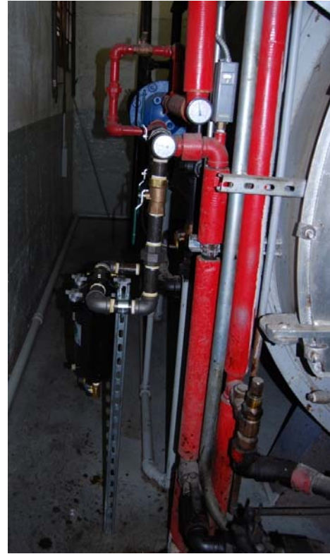
Fitch Installation on Boiler Fuel Line
