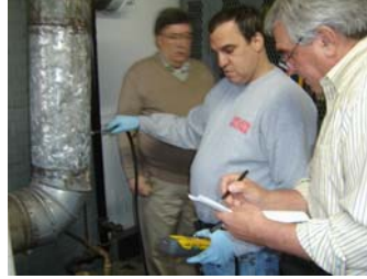
Using UEI Combustion Analyzer – Collect Baseline Data
