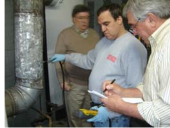
Using UEI Combustion Analyzer – Collect Baseline Data
